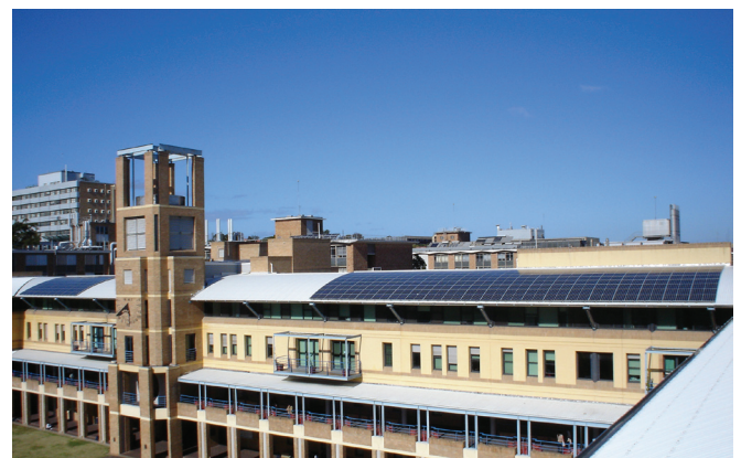
Above: 42-kilowatt (peak power) grid-connected photovoltaic system on the north-facing roof of the Quadrangle building. The photovoltaic cells were developed by UNSW research teams Left: The library building at the University of New South Wales Left: Lowy Cancer Research Centre Project UNSW
